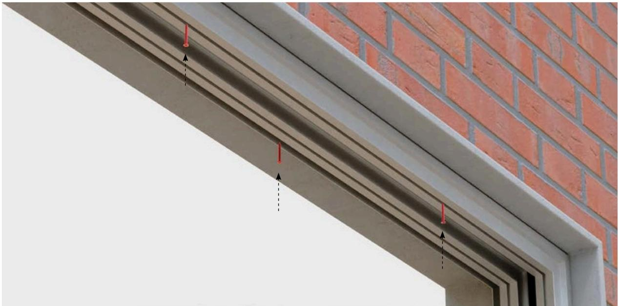
**14** Where possible, fixing points should be on both sides of the frame, in a zig-zag pattern.
